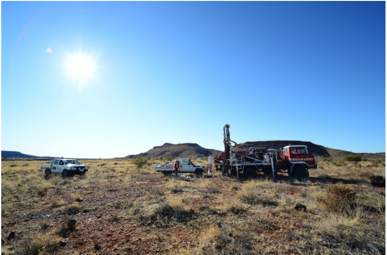
Figure 4. DRX drill rig and support truck located on the Tick Hill Tailings Dam.
