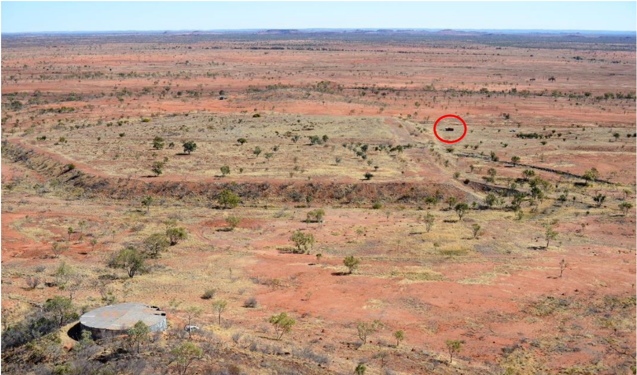
Figure 1. Tick Hill Gold Project Tailings Dam and Tailings Decant Pond (looking West). DRX drill rig and support truck located on decant pond circled in red.
